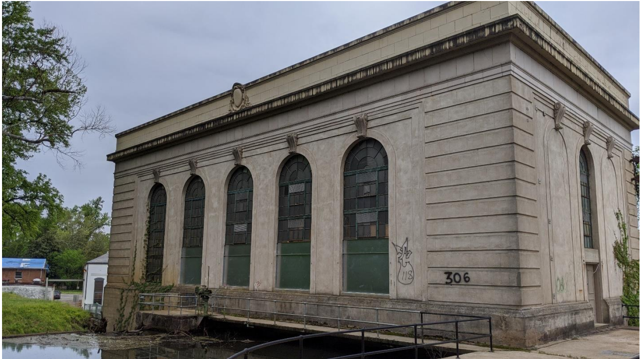
North façade showing the existing blank off panels at the bottom of the windows.
