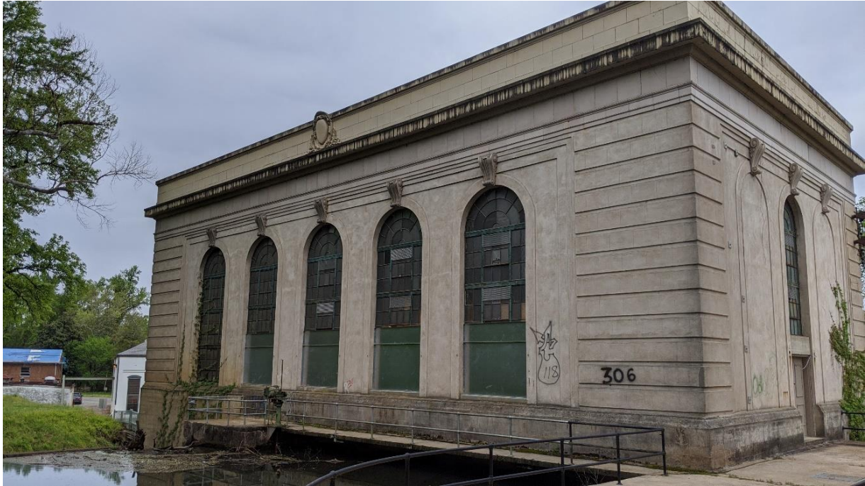
The North façade showing current blank off panels.
