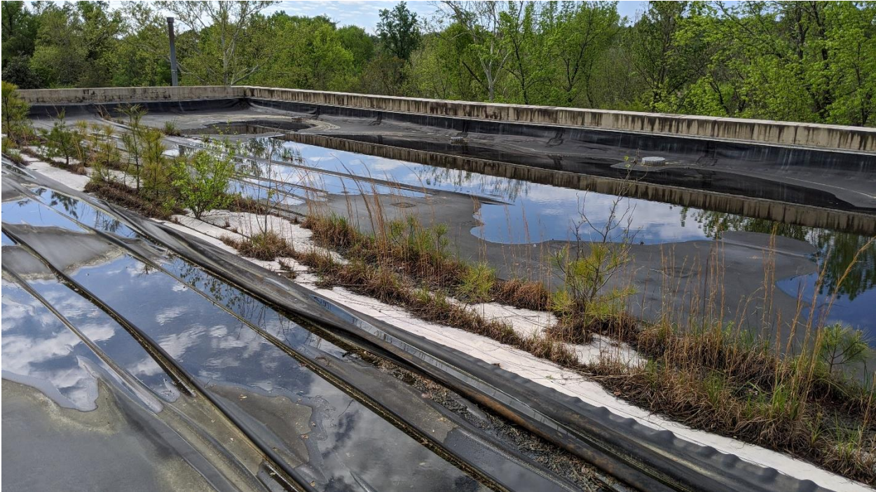
Current roof condition
